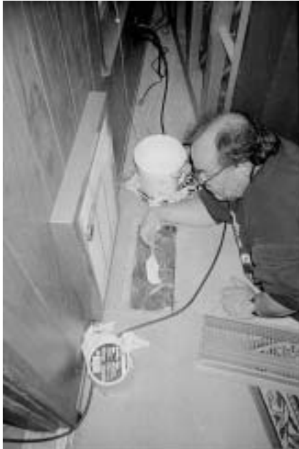
(above) Sealing ducts at air distribution registers with mastic.
